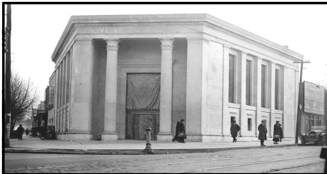
Parkside Trust Company (c1926) SE Corner of Haddon & Kaighn Avenue (see trolley tracks in Haddon Ave) The building later would become a Buten Paint store in the late 1950's (Courier-Post Archives)
